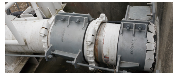
東日本大震災でも通水機能を維持した伸縮可とう管 Flexible expansion pipe that maintained water flow function even after the Great East Japan Earthquake.
