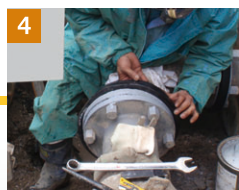
4 Rubber ring installed
