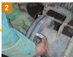
2 Replacement of flange bolts
