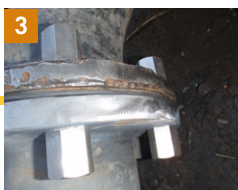
3 Surface preparation & painting
