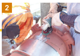
Surface preparation & painting
